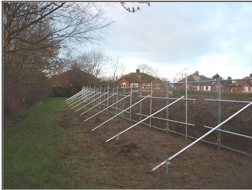
Figure 2- Actual barrier erected on site
